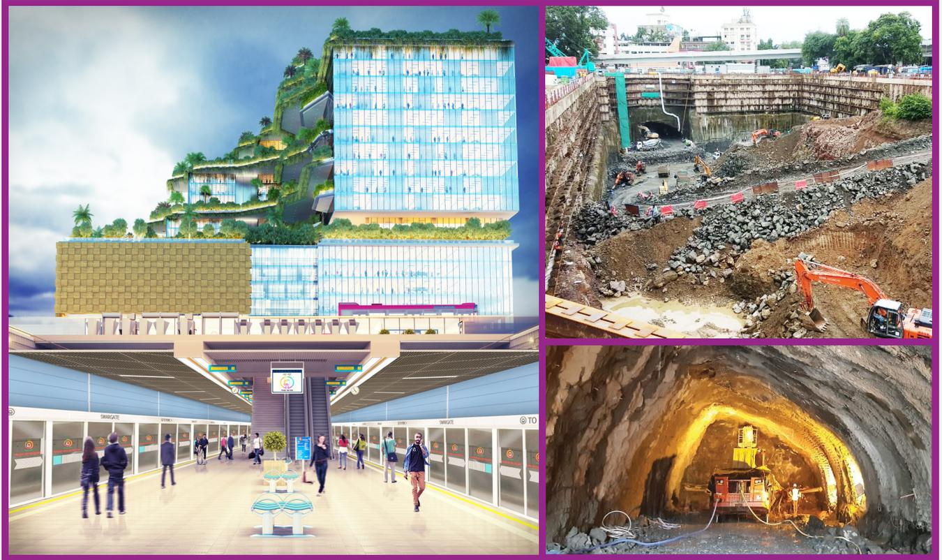
Swargate Multi Modal Transportation Hub (MMTH) excavation comprises of Underground Metro station with multi levels of commercial development above it and MMTH building consisting of 5 levels of underground parking, concourse and upper concourse levels. The total depth of excavation is enormous 28 m approximately.
